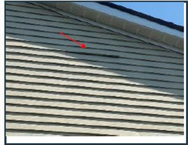
Photo 3: Typical siding lift up
