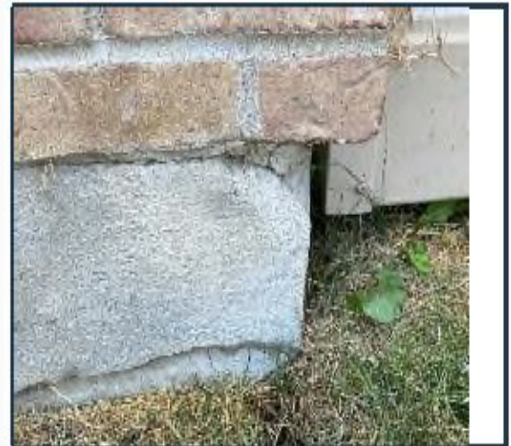
Photo 8: Foundation missing
