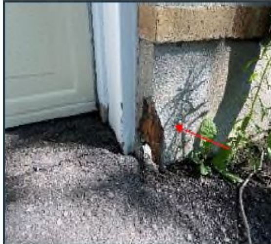
Photo 7: Observed exposed foundation from cracking.
